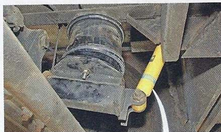
5. The new air bag and Bilstein shock absorber are shown in place on the
